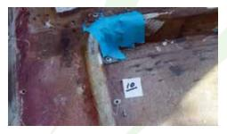
This is what your repair will look like, when your are finished. A little scuffing with some 80 grit paper to knock down any pointed or sharp fiberglass threads, and you are finished with this repair.
