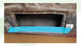
I apply spray glue to all the 2' wide tape as I am installing them. Start at the top and work your way down overlapping about 1/2". It's super important to completely cover the bottom inside the first piece
