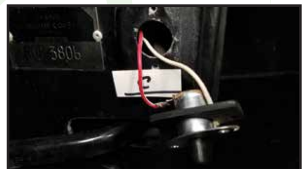
Photo C shows how the ground wire was run through the rubber seal
